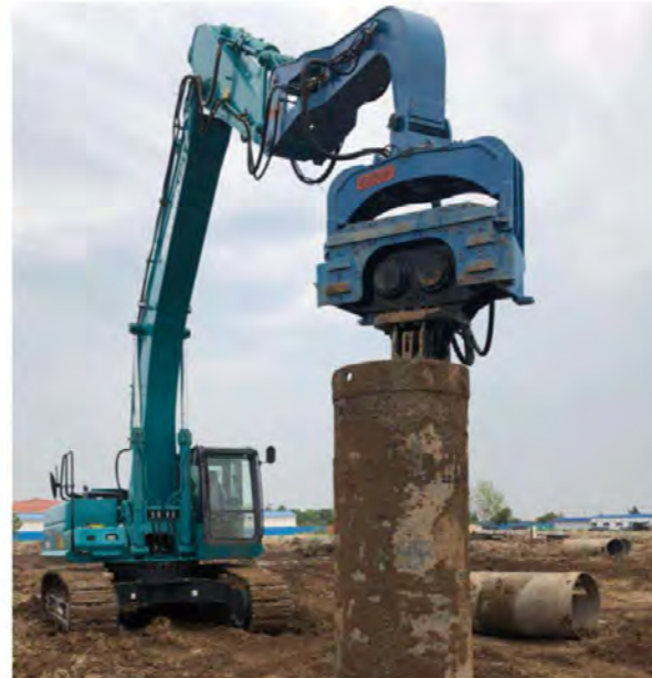
V-400 Casing driving
