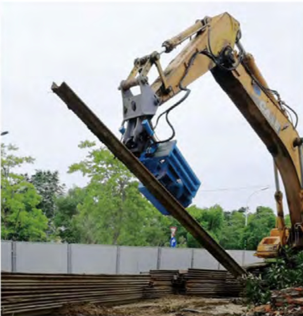
UMS Pile excavating
