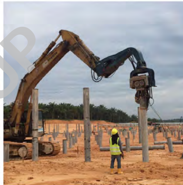
V-250 Pile piling with custom-made clamps
